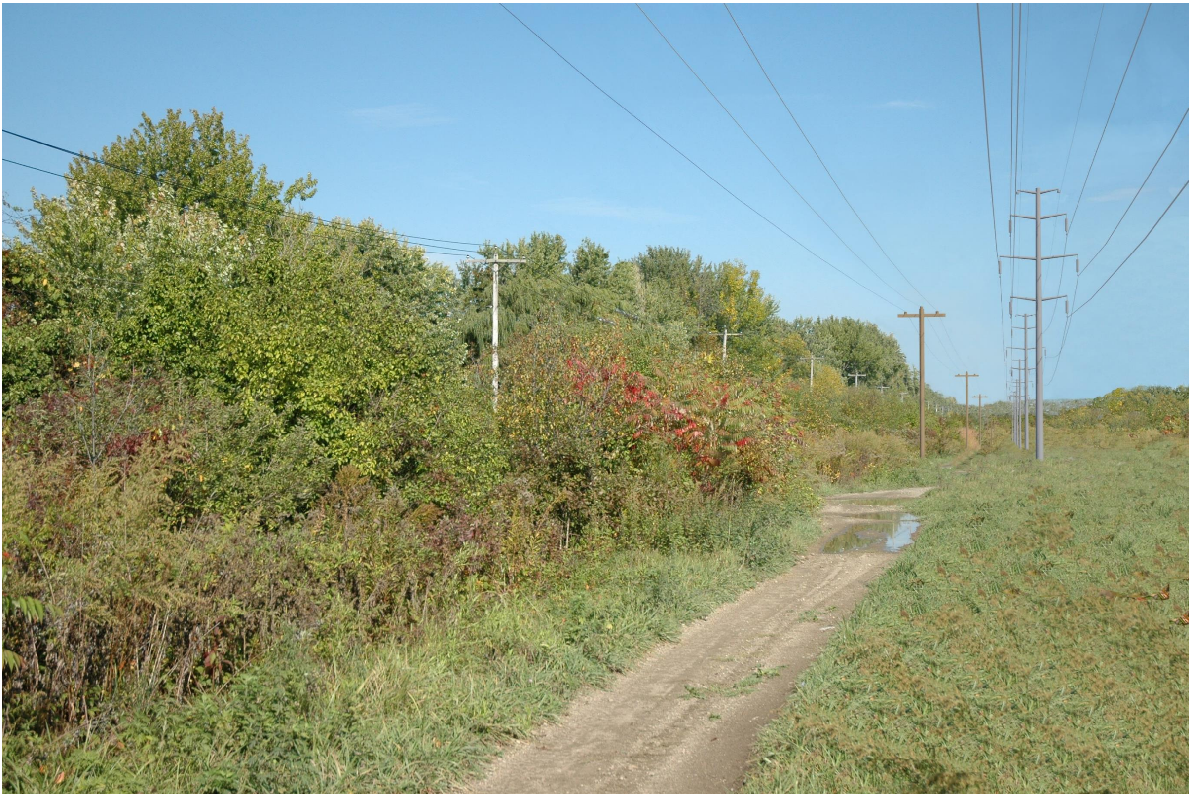
View east. Closest structure to viewer is #129
