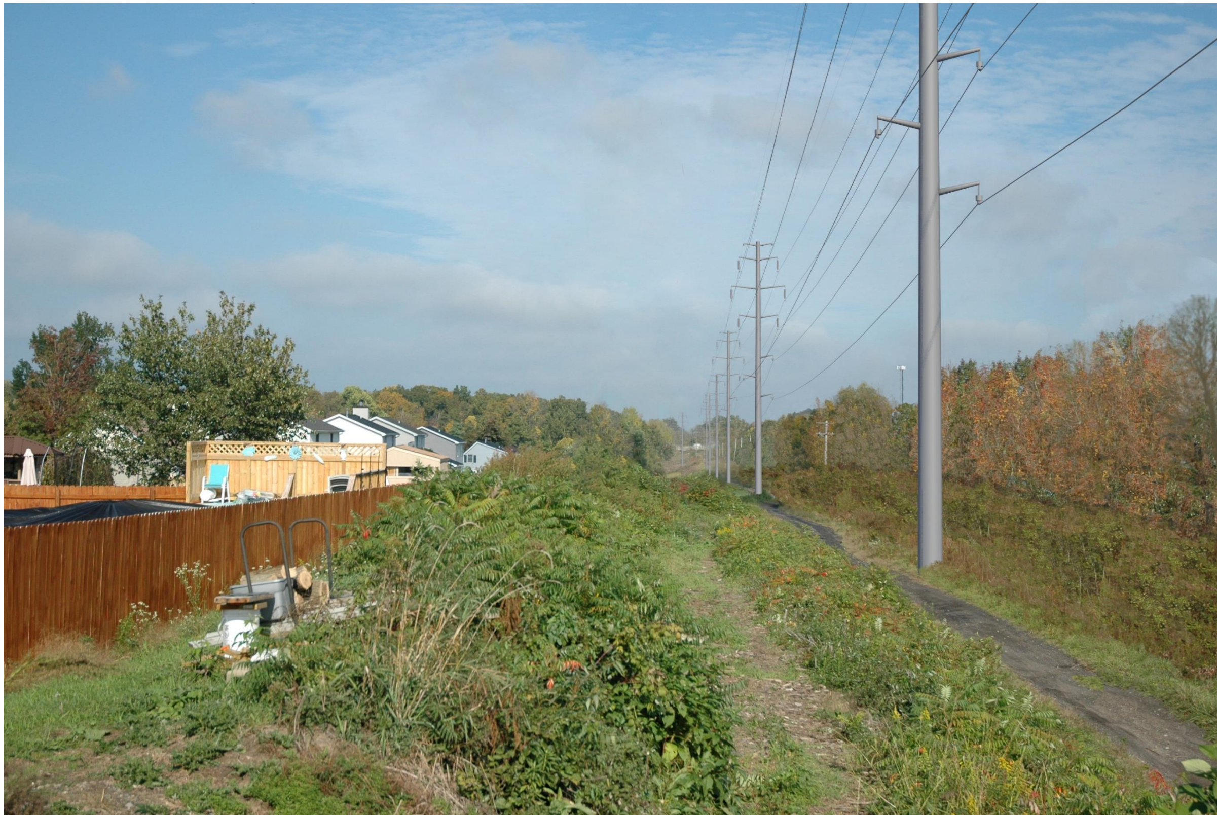
View east. Closest structure to viewer is #161
